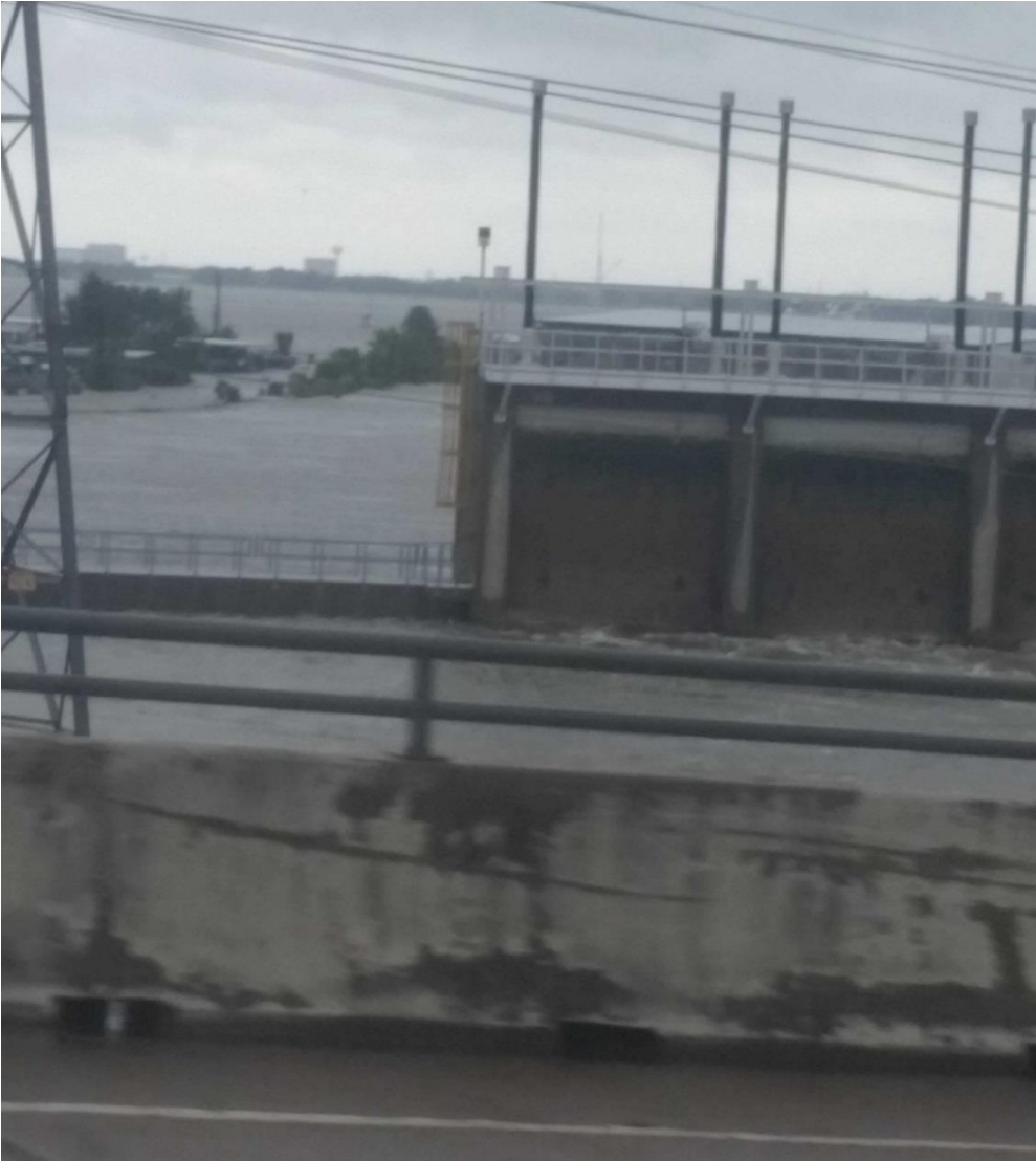
Views of Clear Lake's 2nd Outfall during Hurricane Harvey showing floodgates open with the bottom of the raised floodgates submerged and water rushing beneath.
