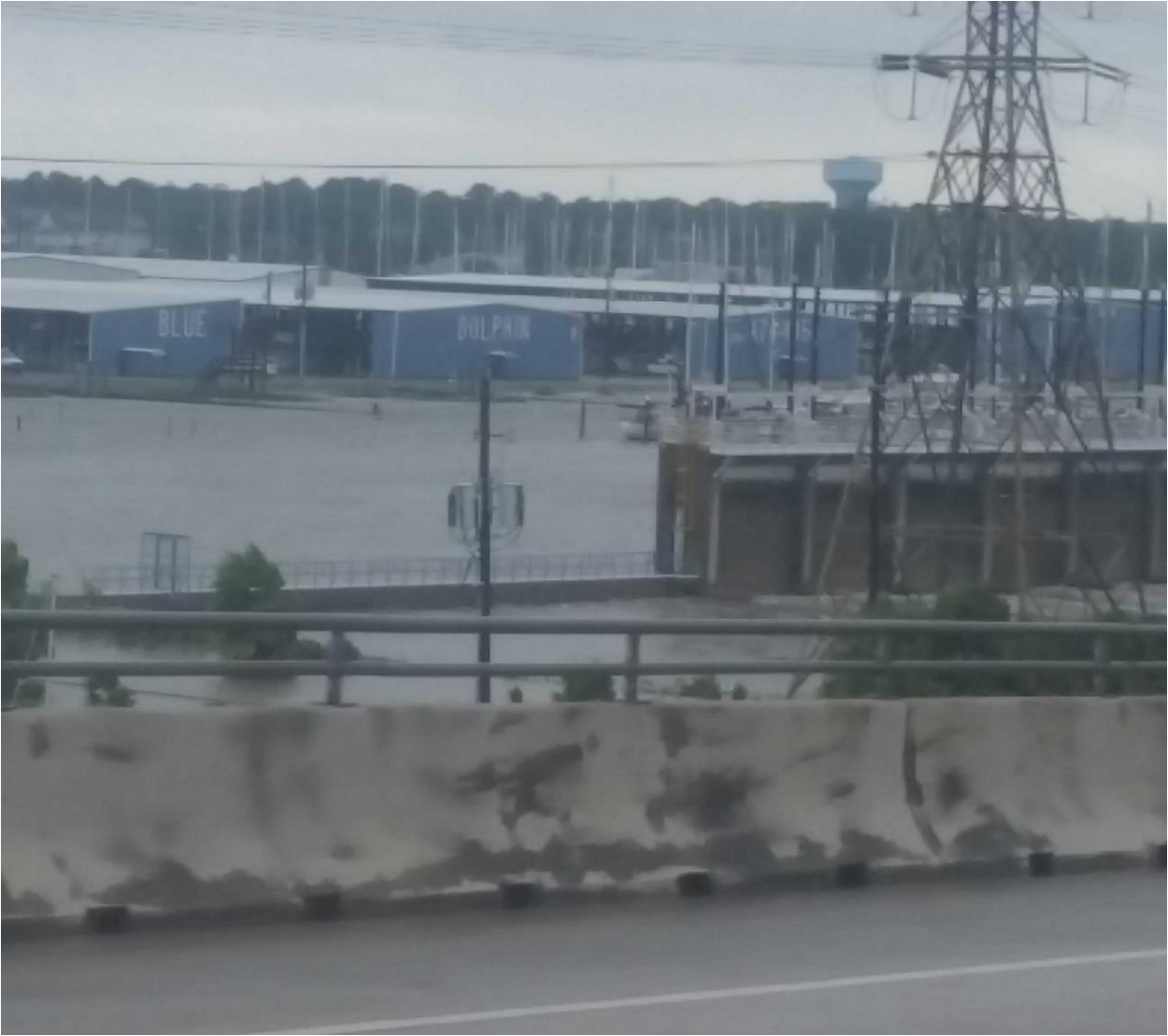
Views of Clear Lake's 2nd Outfall during Hurricane Harvey showing floodgates open with the bottom of the raised floodgates submerged and water rushing beneath.
